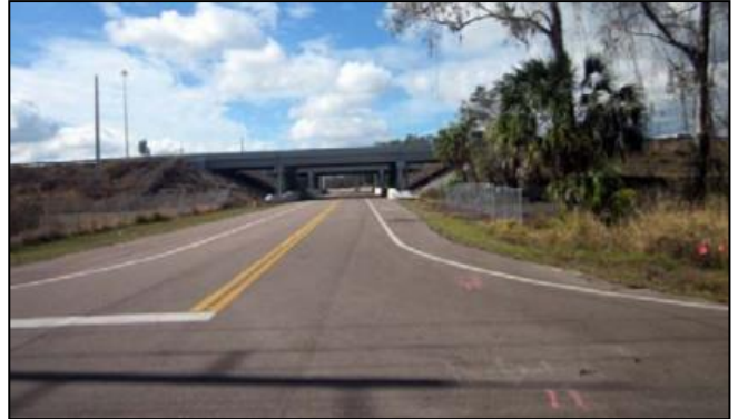
View looking west off 127 th Ave underpass towards Morris Bridge Road
