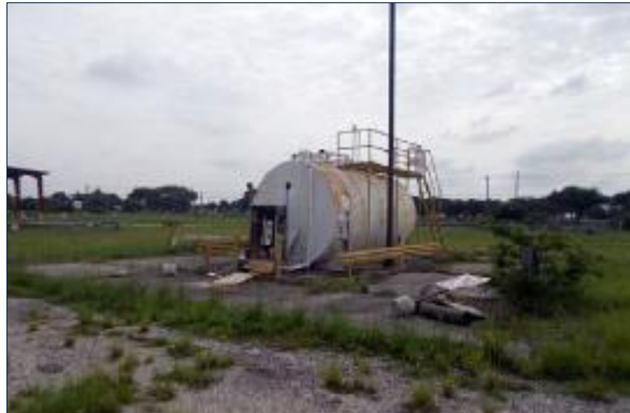
FUEL STORAGE TANK
