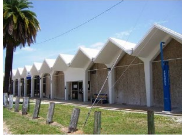
North elevation of Corporate Training Center and access to gated City parking lot
