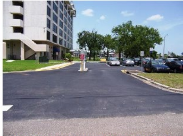
Northerly gated access drive and west and south elevations of Administration Building
