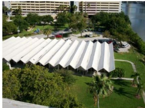
View of the Corporate Training Center roof
