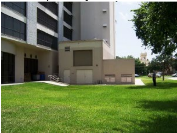
Exterior view of chiller room
