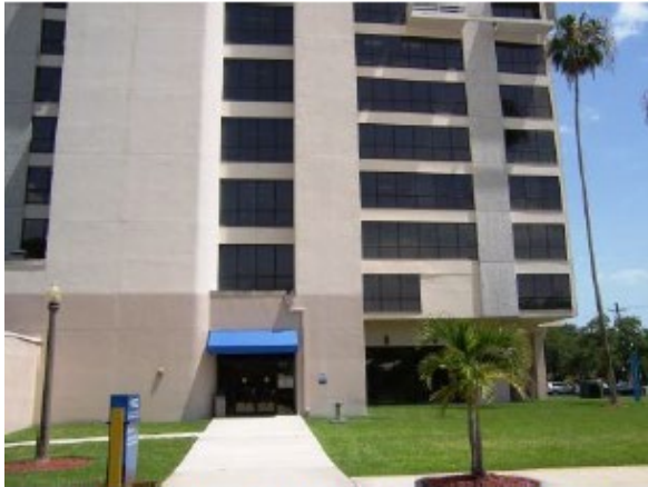
North elevation of Administration Building
