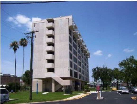
West and south elevations of Administration Building
