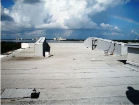
Administration Building roof before renovation
